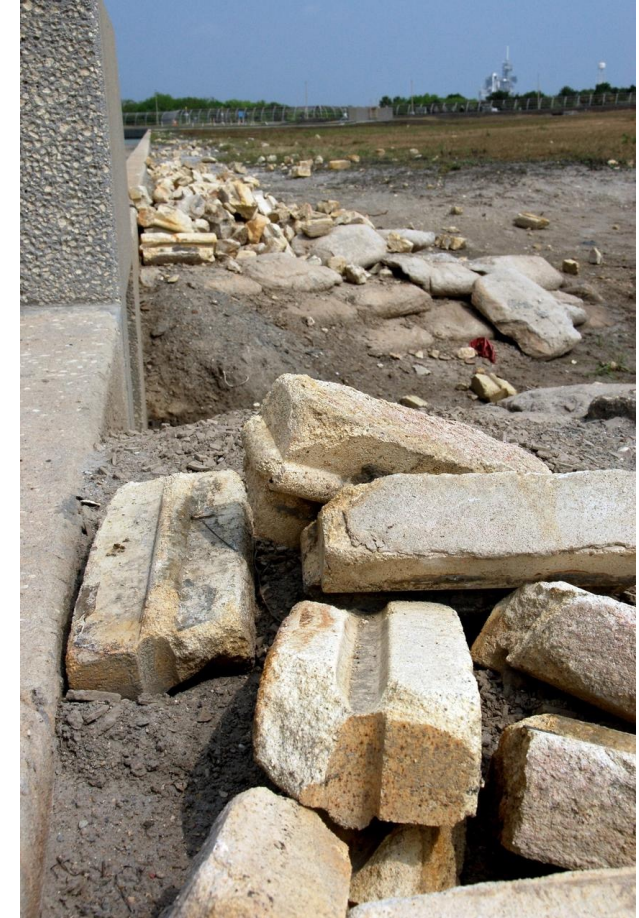
Debris stretches along the perimeter of Launch Pad 39A at NASA's Kennedy Space Center. It is residue from the damage that occurred during the May 31, 2008 launch of space shuttle Discovery.
